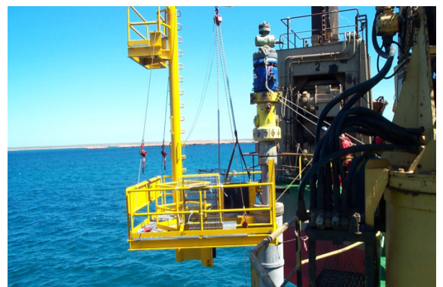
Installation of the topsides structure on the caisson
