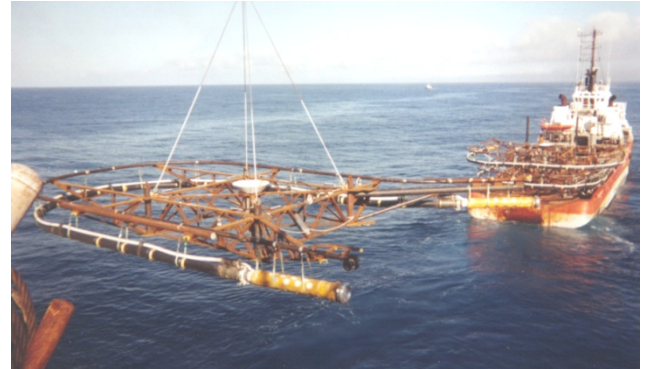
Lifting a frame from the vessel with the rig crane
