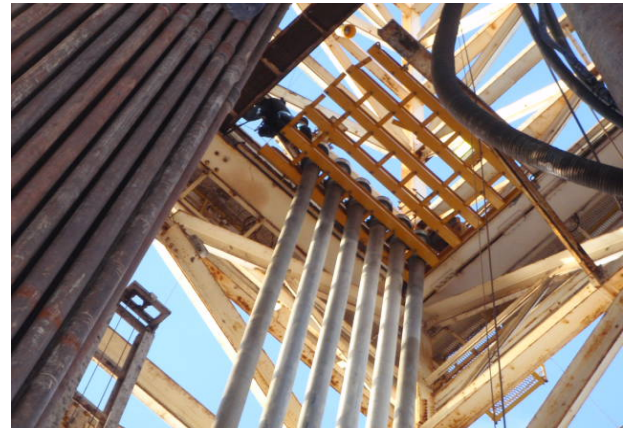
Fingerboard in operation
