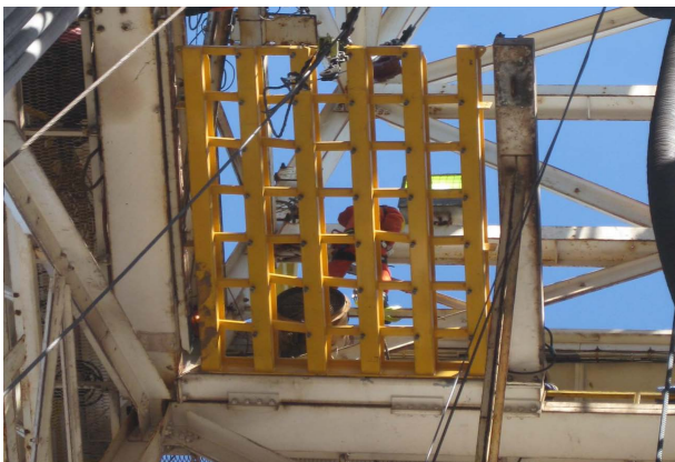
Fingerboard installation using rope access team
