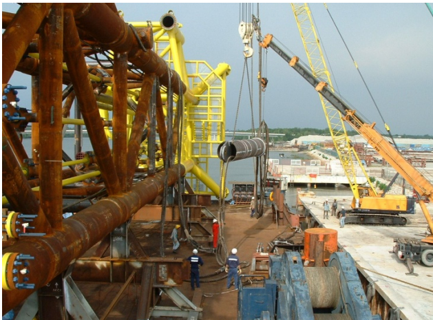
Seafastening of Jacket & Fitting of Lift/Upending Rigging
