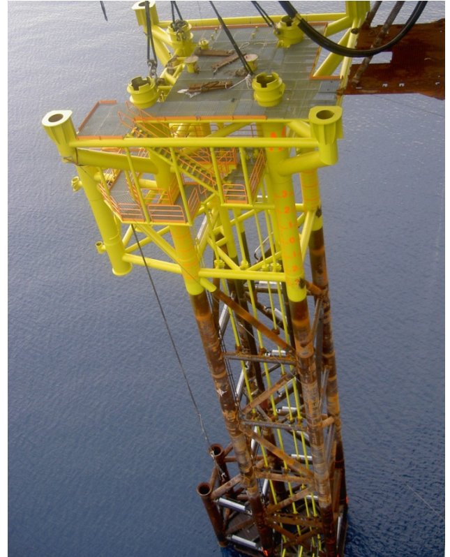
Securing of Jacket to conductor deck prior to lowering to seabed
