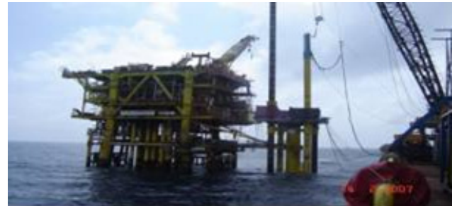
Pile/Conductor installation
