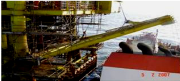
Brace being installed on existing BKC Platform
