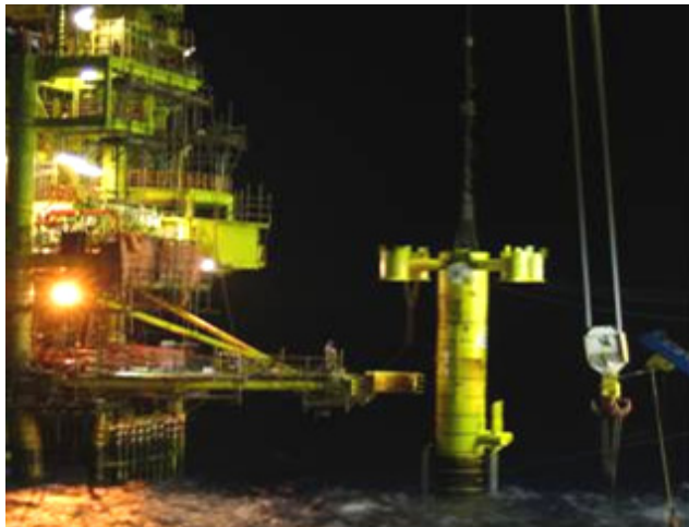
Lifting Monopod into clamp on the end of the brace
