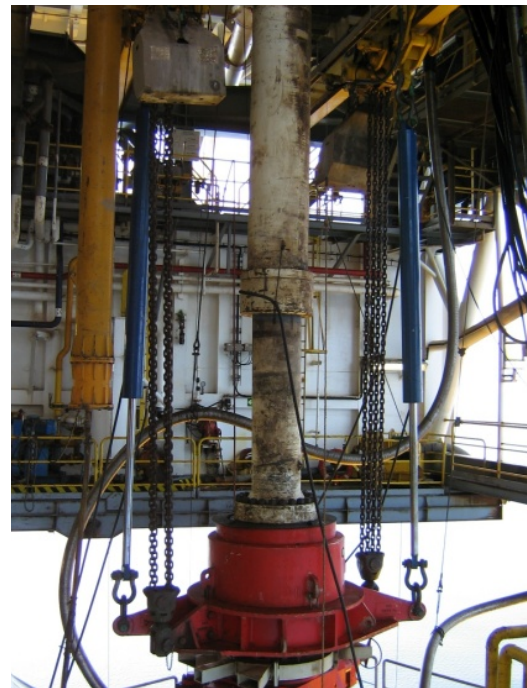
Top Tensioning BOP Crane Installation (System B)
