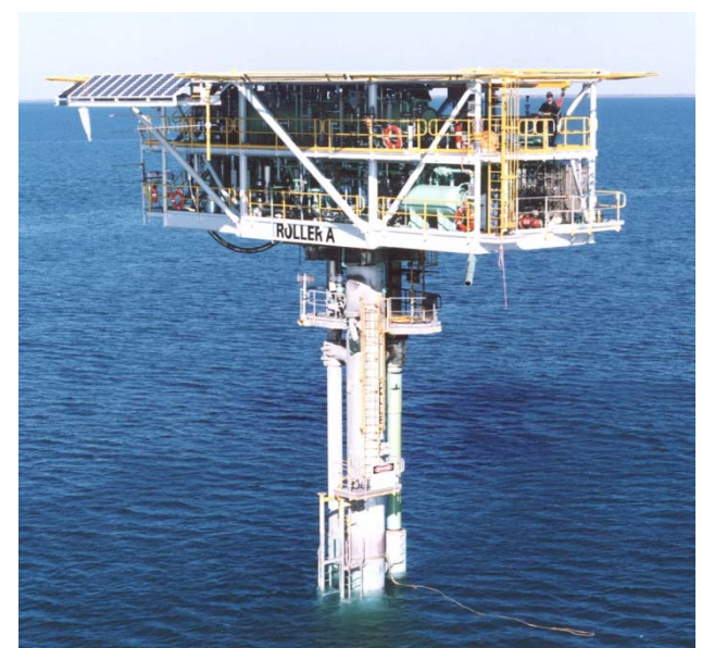
The completed Roller A platform
