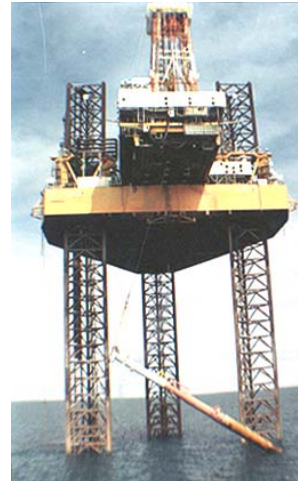
Substructure upending
