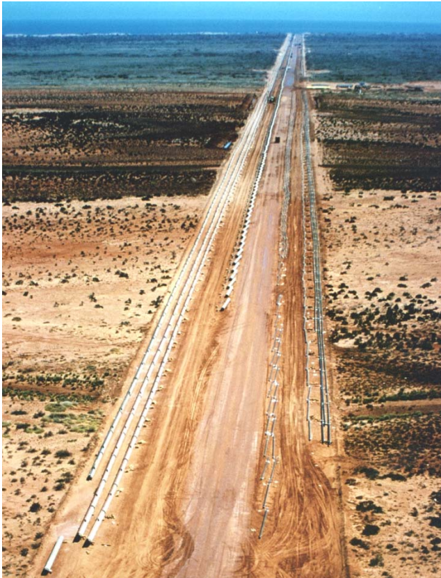
View of the pipeline string site at Tubridgi where the pipeline strings were made up prior to towing to site
