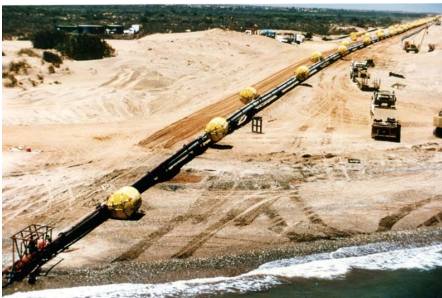
Pipeline bundle with flotation and pull head ready for tow
