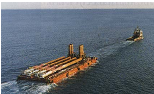
Substructures under tow to location
