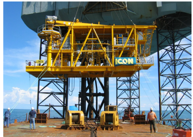
Installation of Linda Topsides
