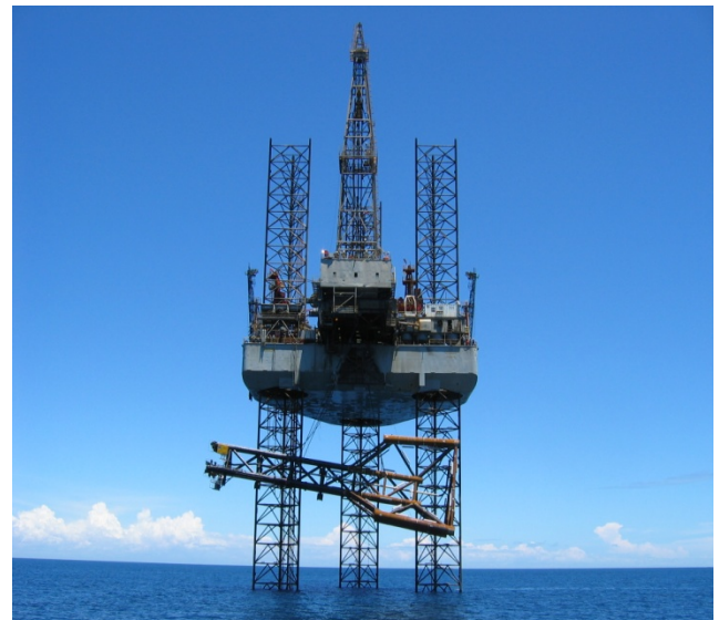
Jacket Immediately after Lift
