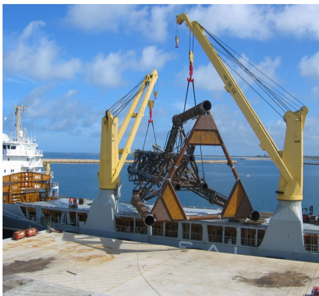
Lifting of Linda jacket onto HLV for transport to Dampier
