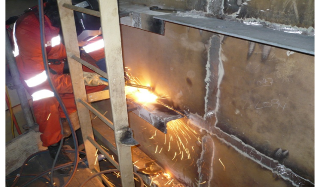
Gas Arc cutting the frames free from the side plate.
