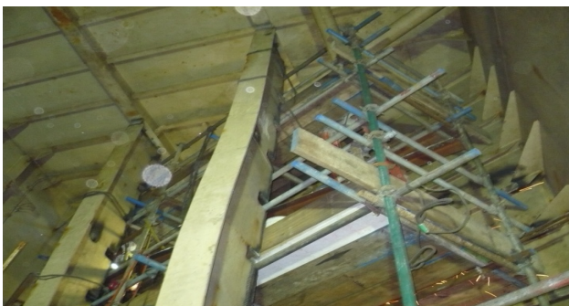
Extensive in-tank scaffolding required.
