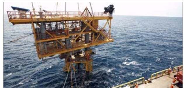
Completed well head platform following separate topsides installation
