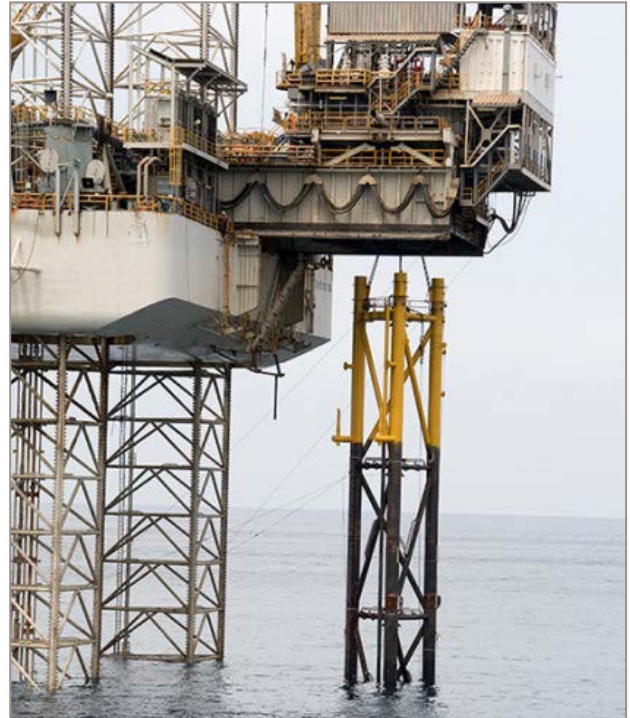
Jacket ready for lowering to seabed
