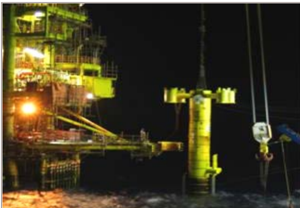
Lifting Monopod into clamp on the end of the brace
