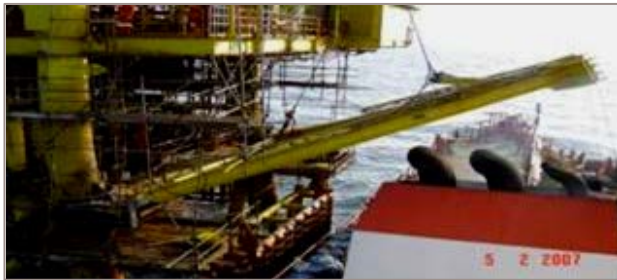
Brace being installed on existing BKC Platform
