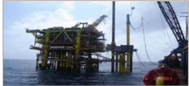
Brace being installed on existing BKC Platform
