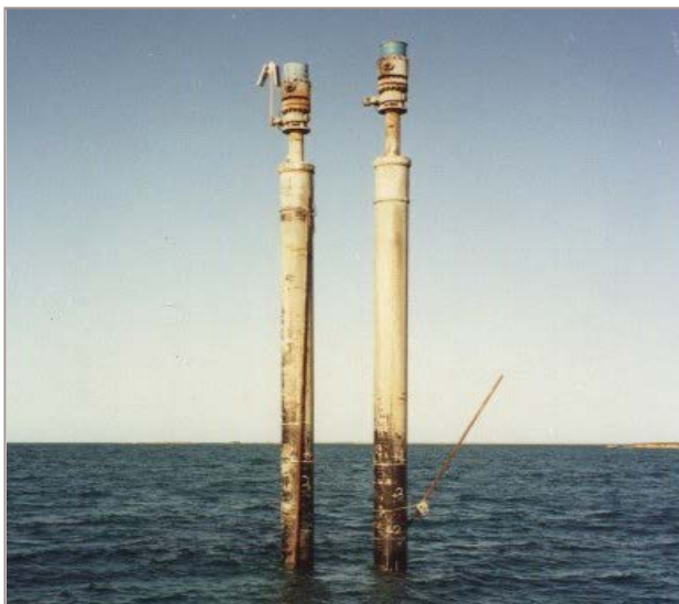
A pair of "Minnowpod" conductors, completed and suspended, awaiting installation of topsides
