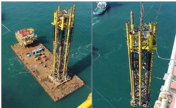
Transportation arrangement and Jacket Lift-off
