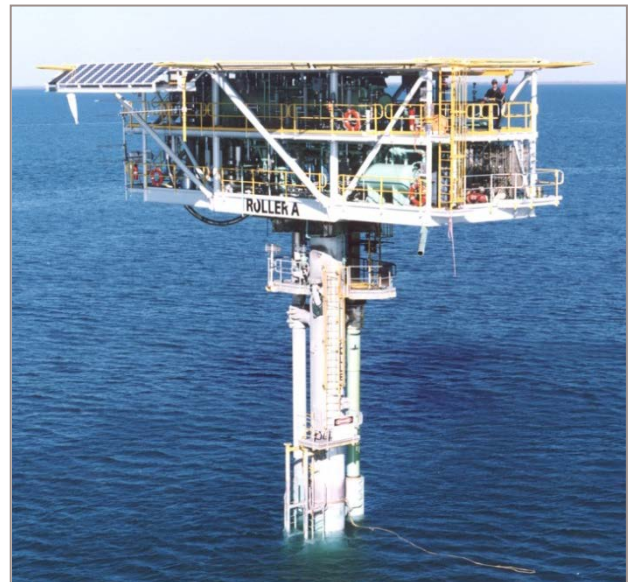
The completed Roller A platform
