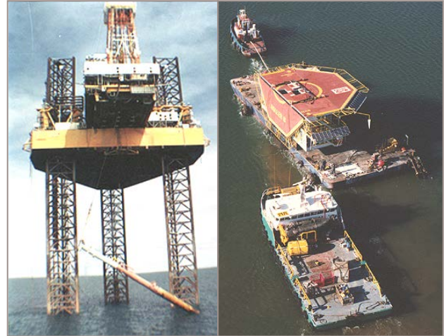
Substructure upending
