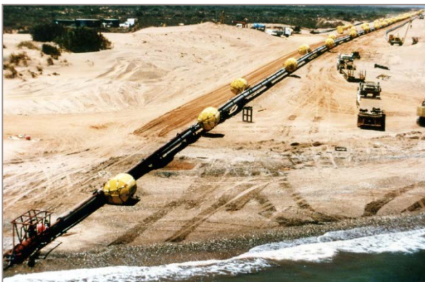
Pipeline bundle with flotation & pull head ready for tow
