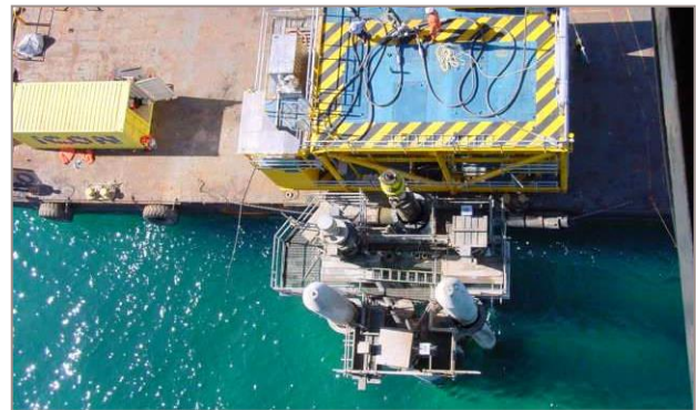
Preparing to lift the topsides
