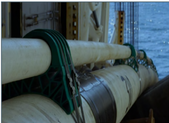
Pipelines - Piggy-Back Installation
