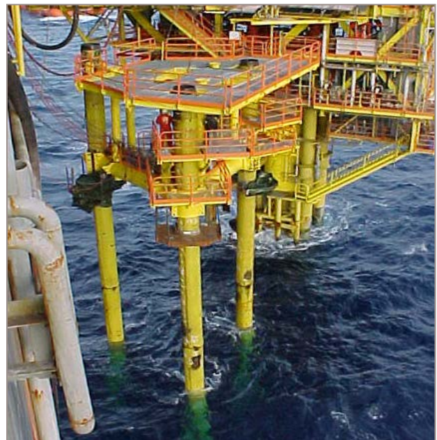
The Completed BKA Annexe Platform
