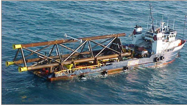
Transport Vessel Standing By, Prior to Lift
