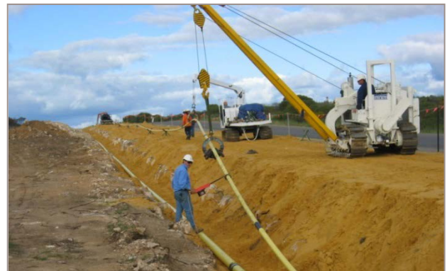
Construction of the carbon steel flowlines from Hovea to Eremia
