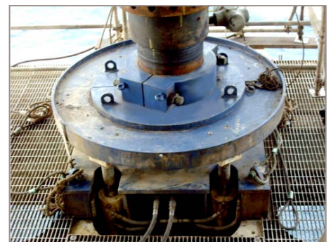
Typical Conductor Gripper Clamp Installation
