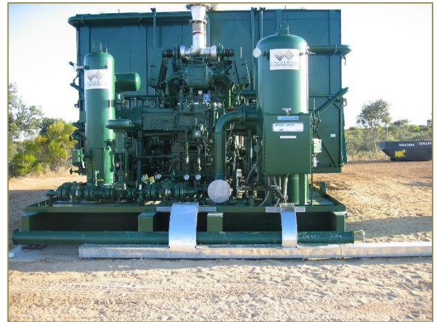
Construction of the XAGGS facilities.
