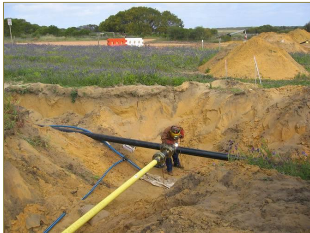
Construction of the XAGGS flowline, which connects the various wellheads to the Xyris gas plant facility.
