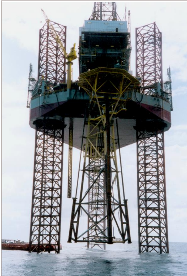
View of the jackup rig Ron Tappmeyer with structure after the lift from the transportation barge
