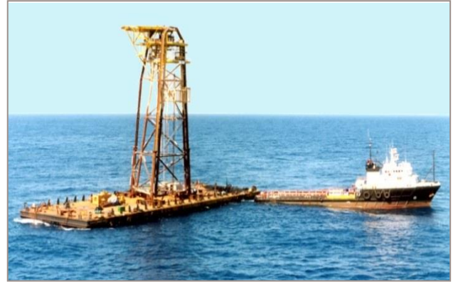
Mooring the transportation barge at site
