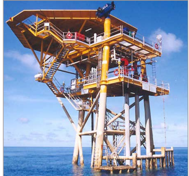
Buffalo Platform as installed
