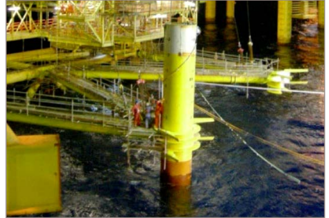
First monopod located into lateral braces
