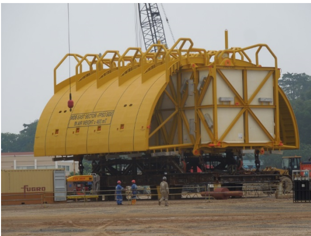
Completed Buoy on Cradle
