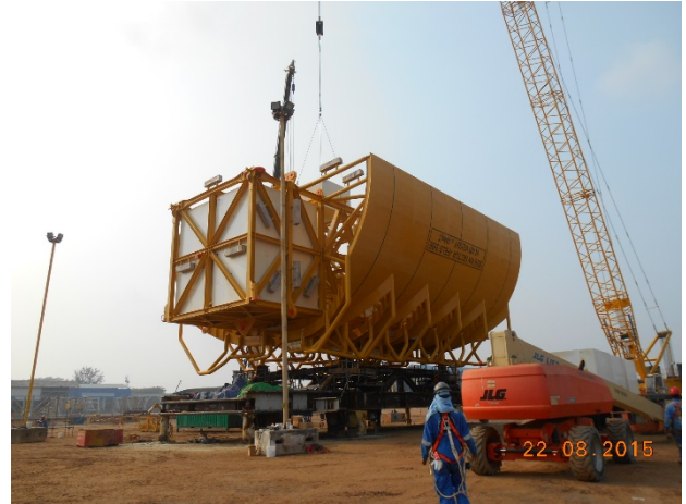
Inverted buoy on cradle for Loading of Syntactic Foam
