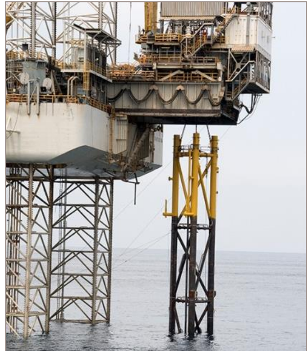
Jacket ready for lowering to seabed
