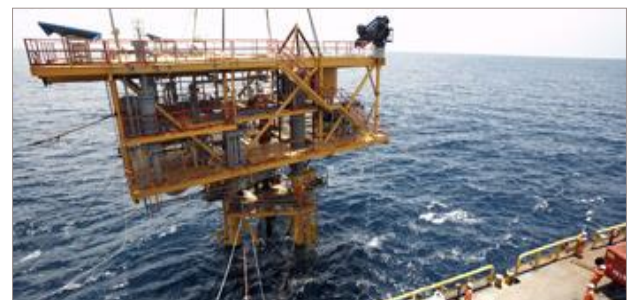
Completed well head platform following separate installation of the topsides
