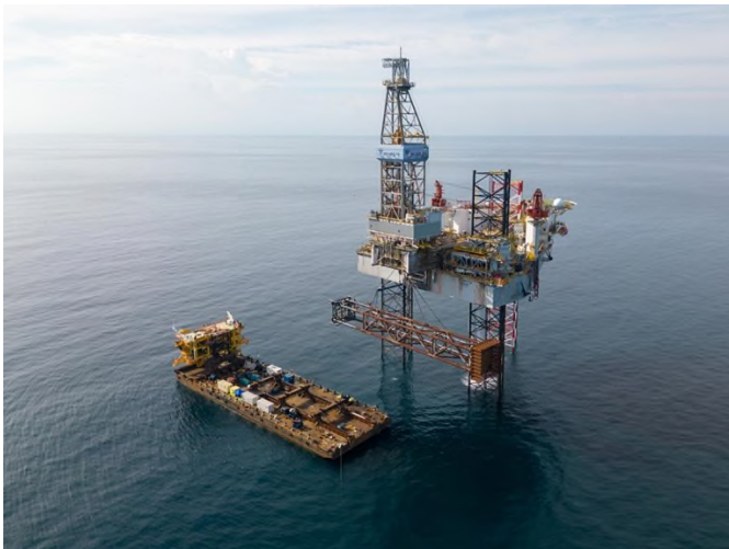
WHP1 being installed using the Jackup Rig
