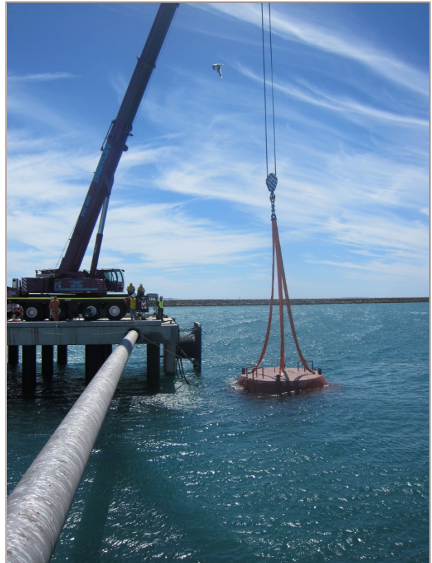
Installing the Buoyant Actuator
