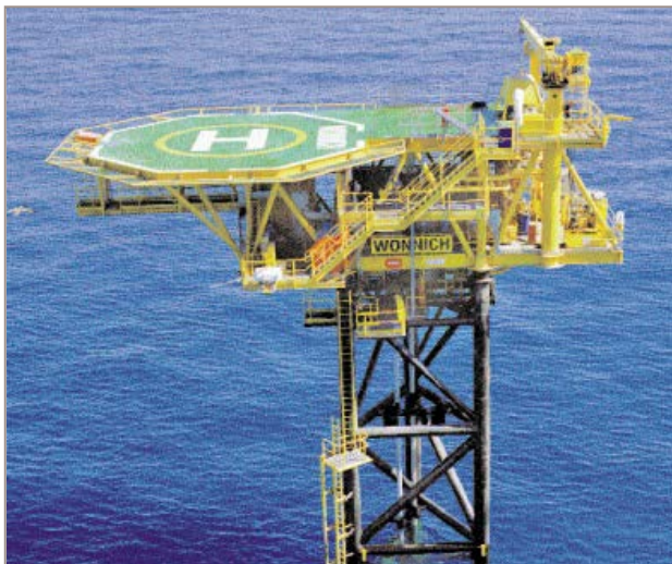
The complete structure was loaded out and transported to site on a single barge
