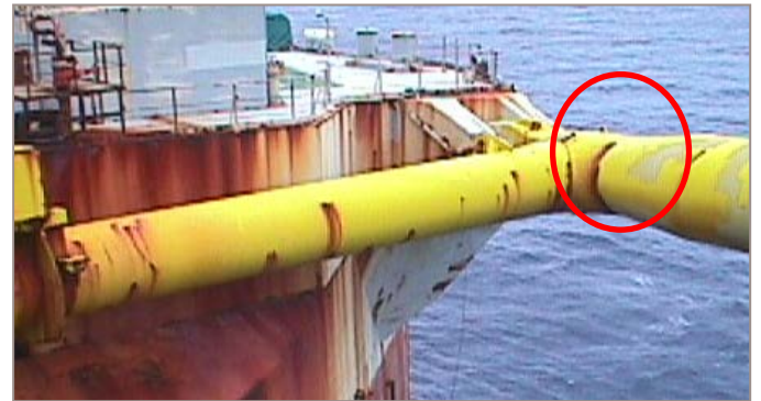
Possible Yoke Cutting Location
