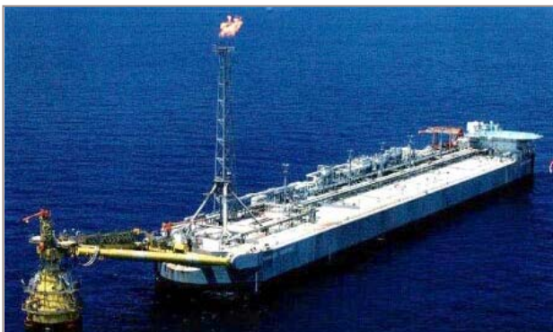
Challis Venture FPSO Connected to RTM
