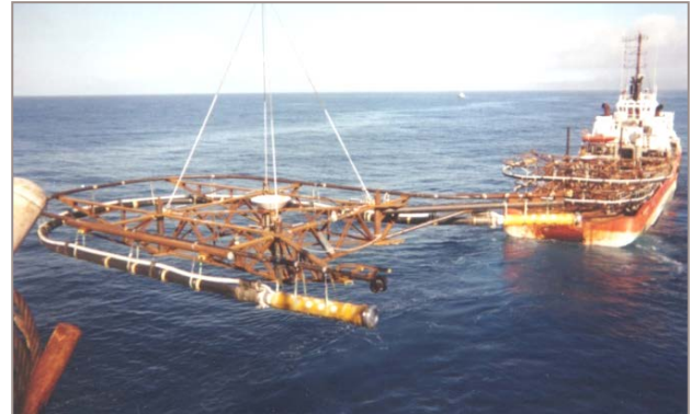
Lifting a frame from the vessel with the rig crane
