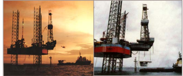
Dawn before topsides lift-off. Mooring and lift takes less than 4 hours
