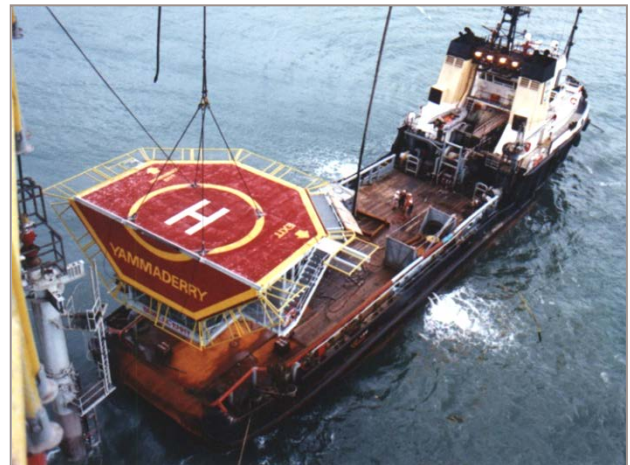
Yammaderry Topsides Installation
