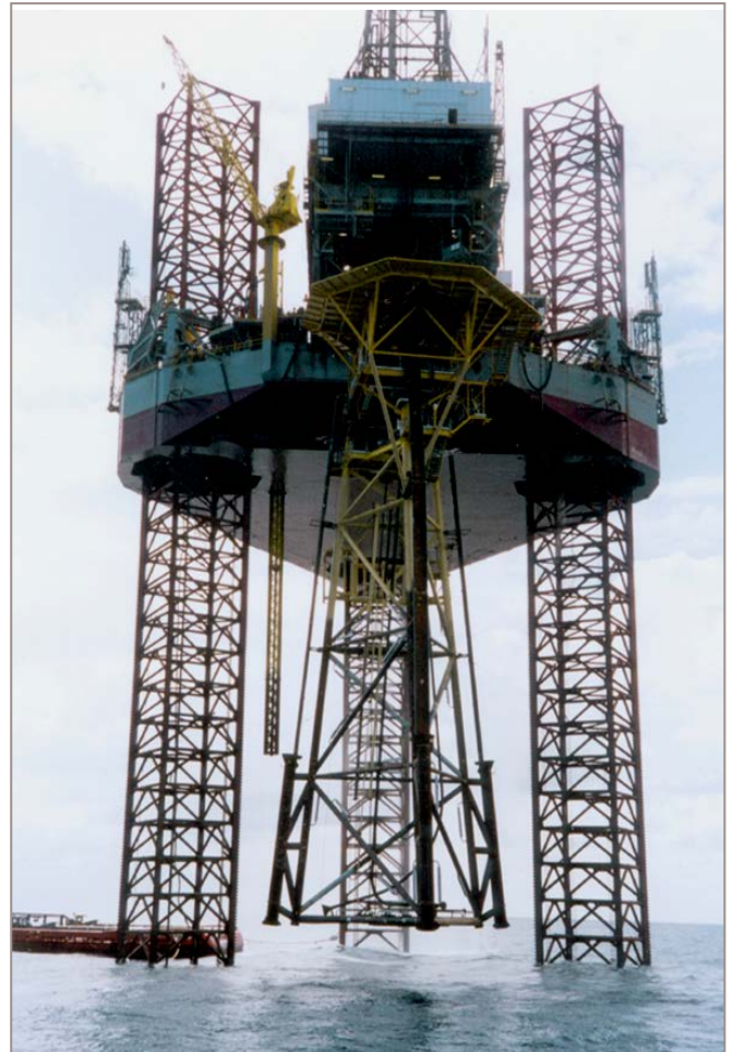
View of the jackup rig Ron Tappmeyer with structure after the lift from the transportation barge
