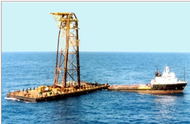
Mooring the transportation barge at site
