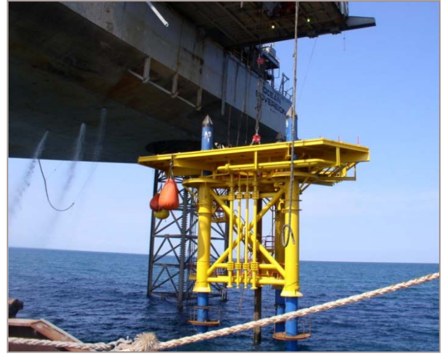
STS Stabbed over 30" Conductors. Production Module not yet installed
