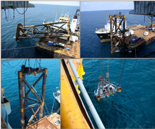
TTS Up-Ending on Barge and Installation onto
