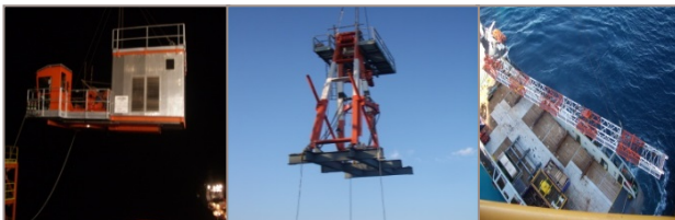
Lifting the main crane units onto WHP
