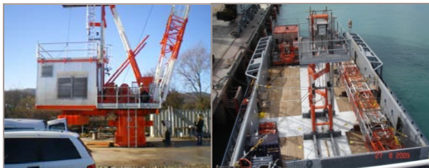
Trial assembly shore side / Sea fastening for
