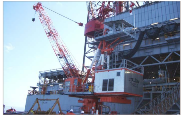
Blacktip crane installed and tested
