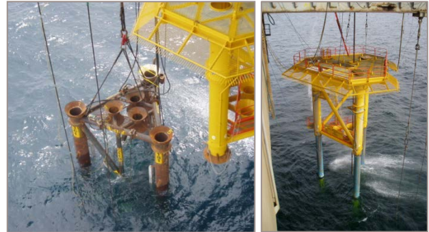
TTS lowering to seabed
