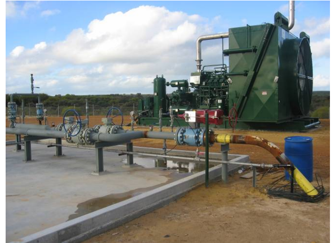
Construction of the XAGGS Flowline Pig Receiver and Xyris Gas Compressor tie-ins
