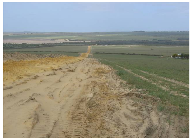
Completed XAGGS flowline with the Xyris South field in the background
